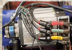
RELIABLE HYDRAULIC SYSTEM
